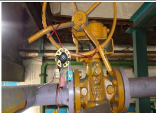
Energy Isolation Arrangement for Valves
