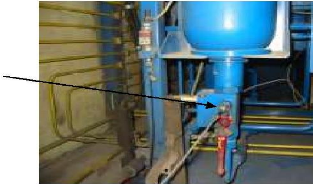
FIGURE- 4: ARROW IN THE PICTURE IS SHOWING MINIMESH POINT
