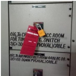
Electrical Energy Isolation Arrangement
