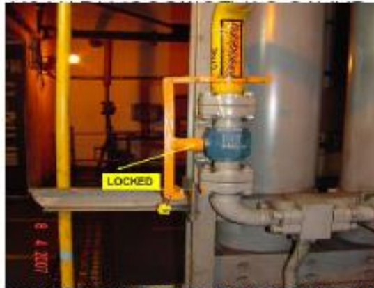
Arrangement made to lock hydraulic line ball valve at HSM
