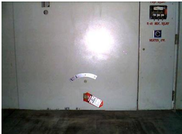
Electrical Energy Isolation Arrangement
