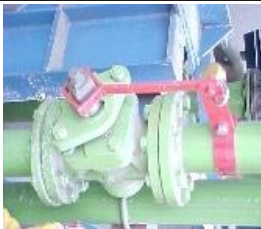
Energy Isolation Arrangement for Valves
